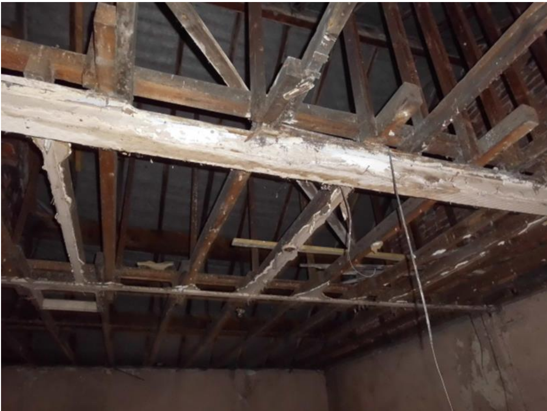
Photo 6: Roof on second floor
